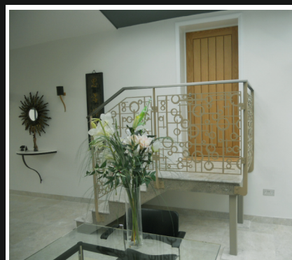
Laser cut, brass stair bannister and railings
